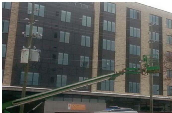
Employees working near power lines risk exposure to electrical hazards. Employers should take precautions to eliminate the hazards.
