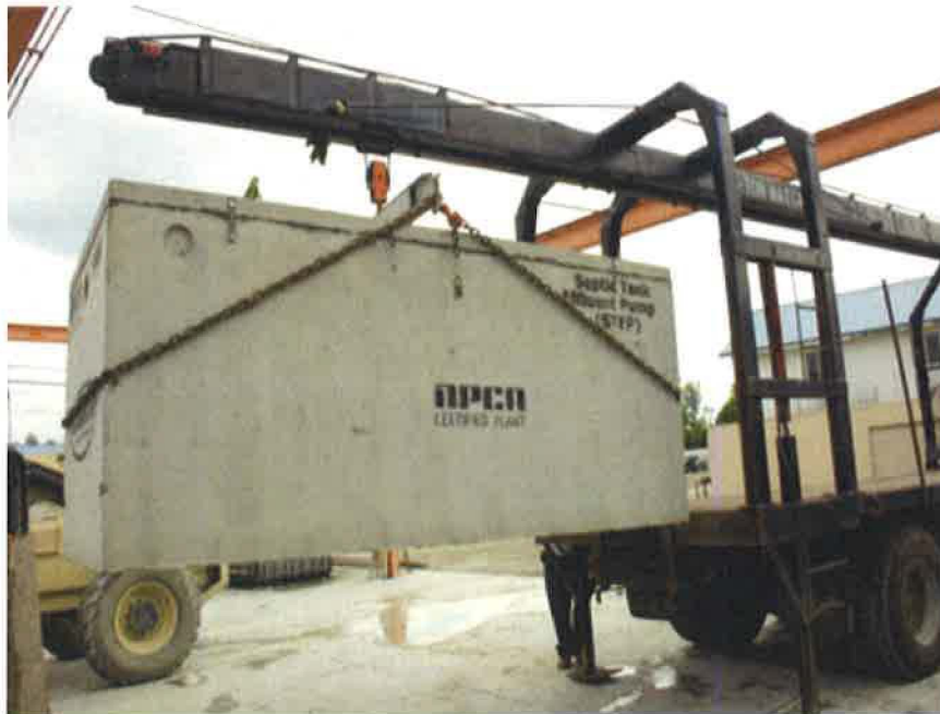
Photo 3: Septic Tank Delivery Rig
