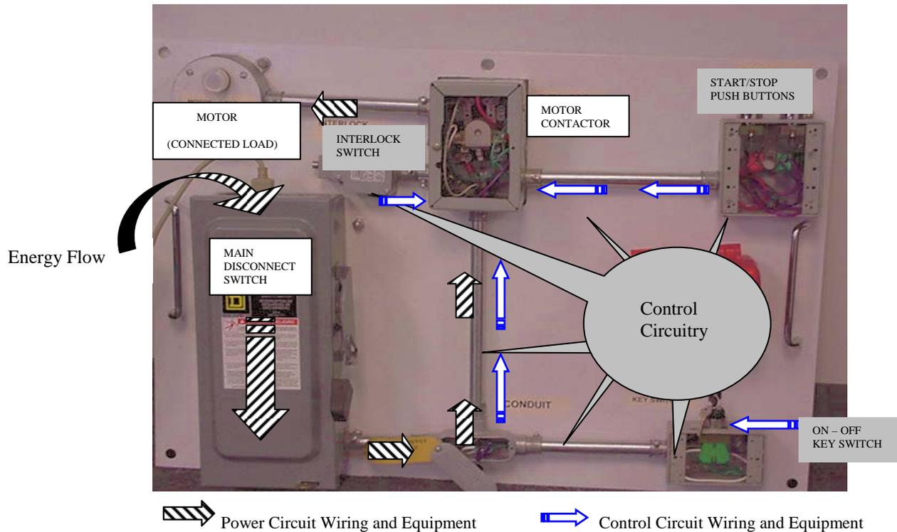
Motor system components may be, in practice, hundreds of feet apart from each other. Thus, the electrical enclosures and conduit may also be subjected to and affected by physical damage, vibration and potentially corrosive and invasive environments.
