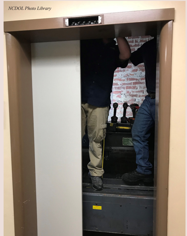
Crews from Bar Construction and Elevator Specialists of Carolina install a digital operating system on the elevator in the Labor Building.
