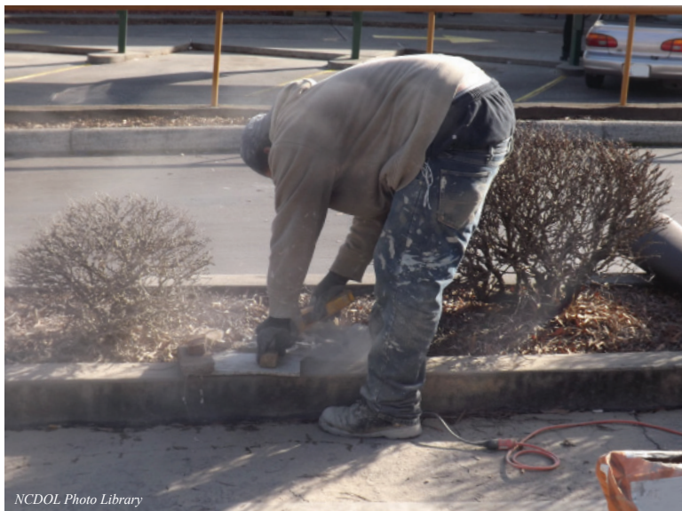
A construction worker creates dust containing silica while cutting through concrete. Exposure to respirable silica dust can cause silicosis, a deadly lung disease.
