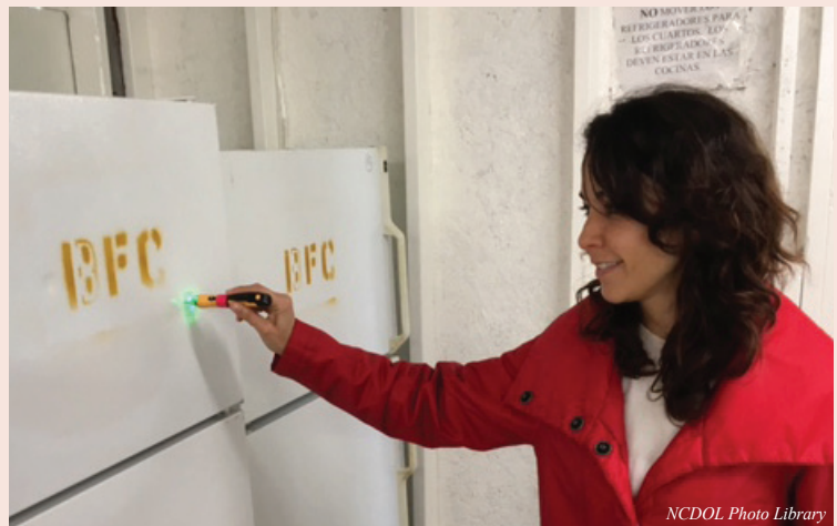
ASH inspector Johana Ramirez uses a tester to check the electricity of a refrigerator at a migrant camp in Nash County.
