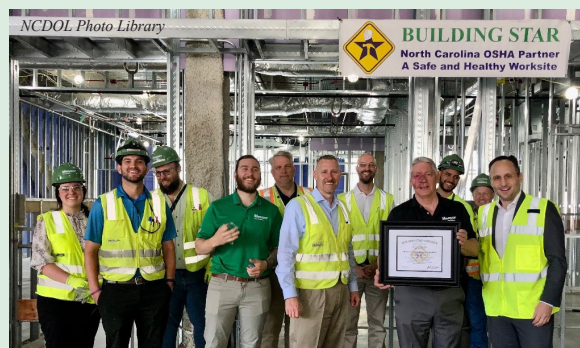
Labor Commissioner Josh Dobson presents the Building Star award to the Messer Construction Co. project team at the Cabarrus County Courthouse expansion worksite.
